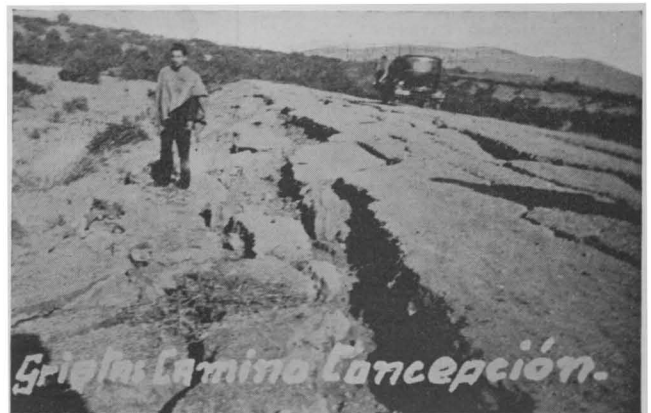
FISSURES IN THE ROAD CAUSED BY THE EARTHQUAKE — NEAR CONCEPCION
