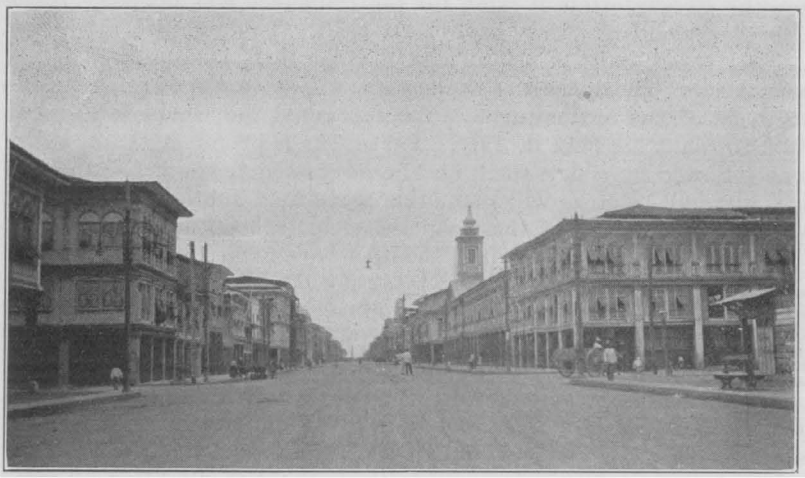
A STREET IN GUAYAQUIL BEING PAVED BY THE AMERICAN ASPHALTING CO.
