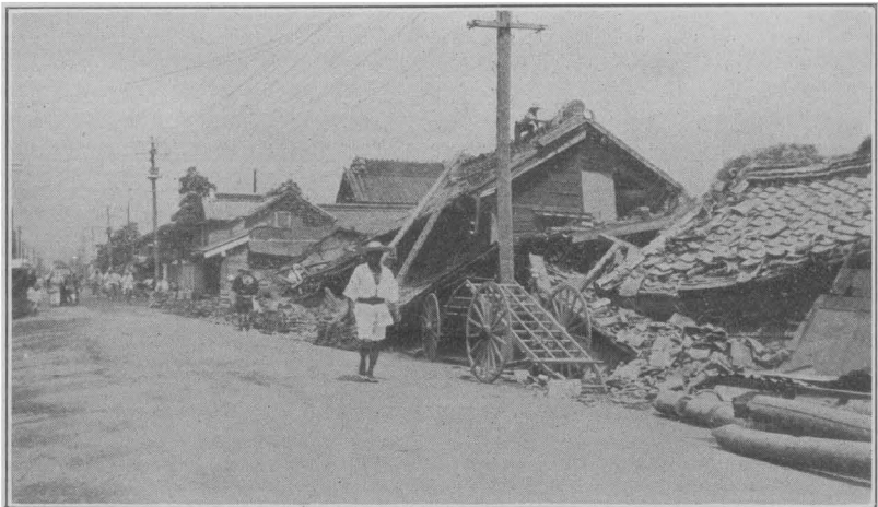
HOUSES THROWN DOWN BY THE EARTHQUAKE IN THE SUBURBS OF TOKYO, BUT UNTOUCHED BY FIRE
