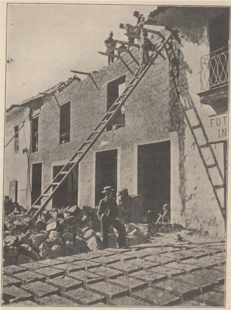
REBUILDING THE MISSION HOUSES IN CUZCO The adobes (mud bricks) are seen drying in the foreground
