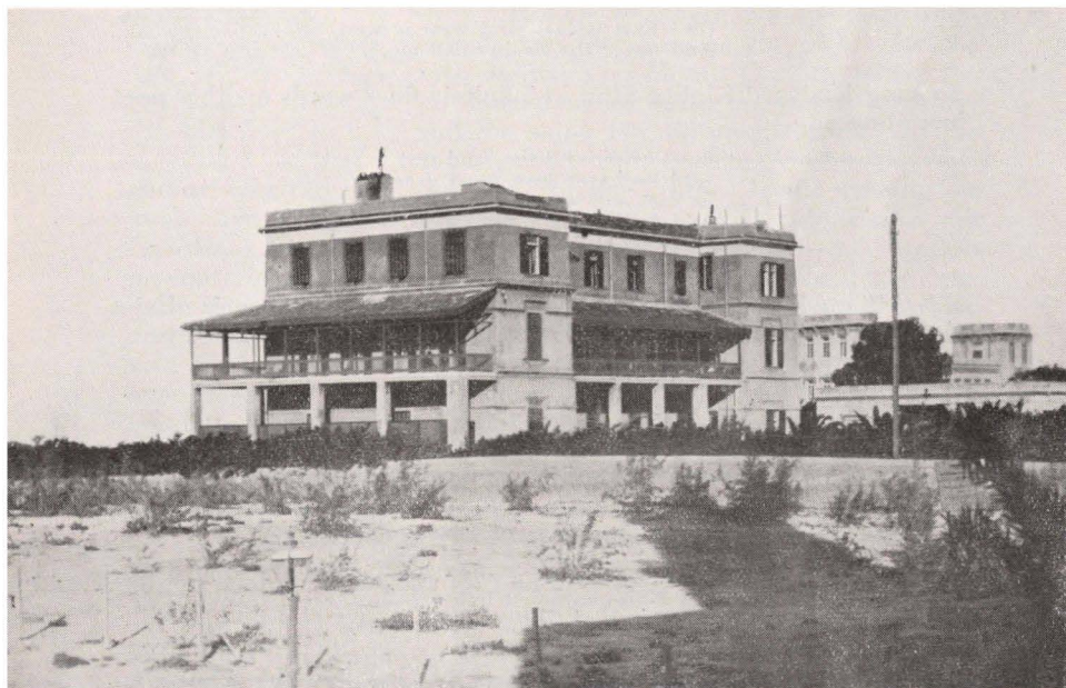
A VIEW OF FAIRHAVEN FROM THE NORTH-WEST.
